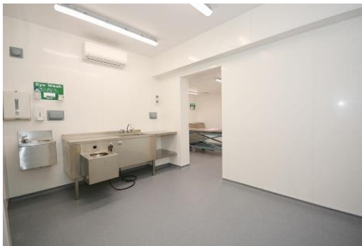
Good standard of preparation area
